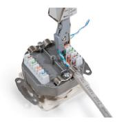
or T568B. Punch down wires with LSA-tool.
