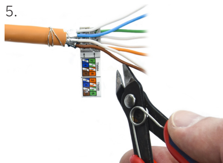
Trim the wires flush with the wire manager.
